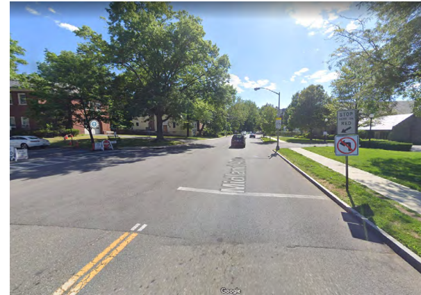
Advance stop bar in Bronxville, NY on Midland Avenue makes it easier for the stop-controlled Palumbo Place approach to enter Midland Avenue. (Source: Google Maps)
