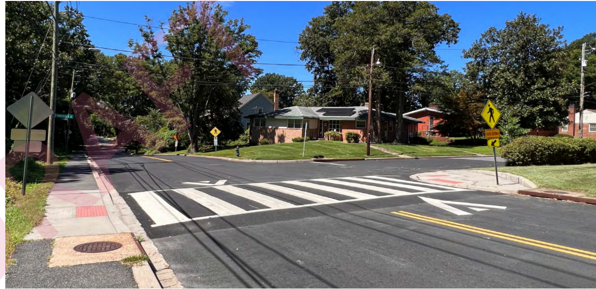
Raised crosswalks, such as this one in Silver Spring, MD, offer two benefits: a high-visibility crosswalk and a speed bump.
