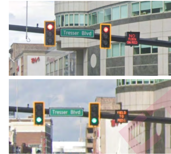
LED Blank-out Signs with variable messages indicate No Turn on Red restriction during leading pedestrian interval and clearly indicates “Yield to Peds” during green interval. (Source: Google Maps Street View)
