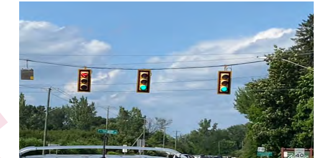
Figure 11. A red left-turn arrow prohibits left-turns during the through movement phase
