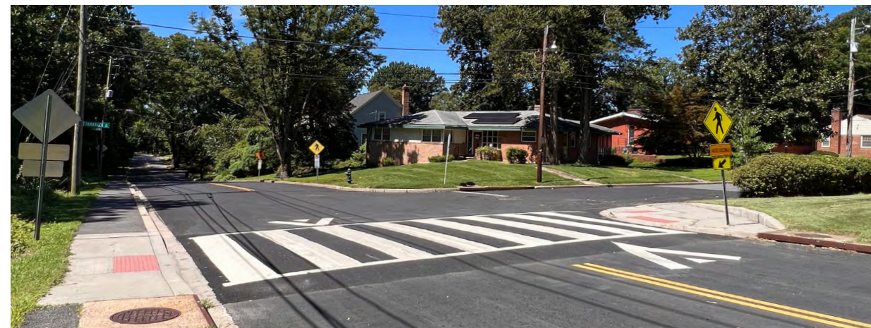
Raised crosswalks, such as this one in Silver Spring, MD, offer two benefits: a high-visibility crosswalk and a speed bump.
