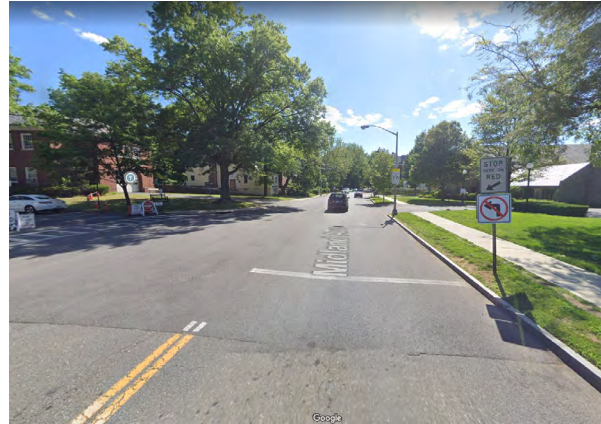
Advance stop bar in Bronxville, NY on Midland Avenue makes it easier for the stop-controlled Palumbo Place approach to enter Midland Avenue. (Source: Google Maps)
