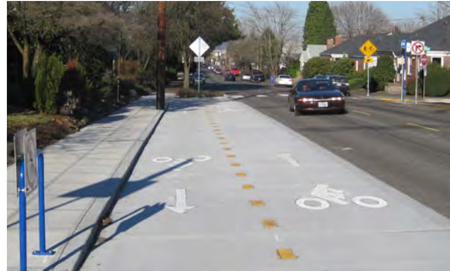
Figure 6. A raised two-way cycle track in Portland, OR
