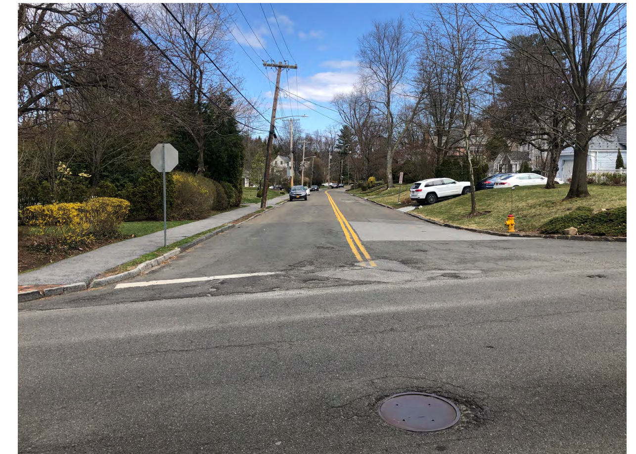
The visibility and speeding concerns at the intersection of Fox Meadow Road and Crane Road could be mitigated by an all-way stop and a raised crosswalk connecting to the existing sidewalk.
