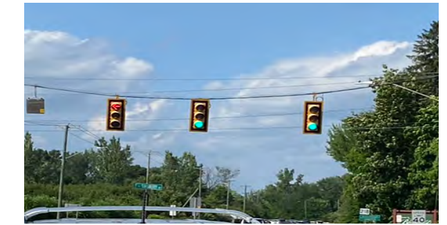
Figure 9. A red left-turn arrow prohibits left-turns during the through movement phase
